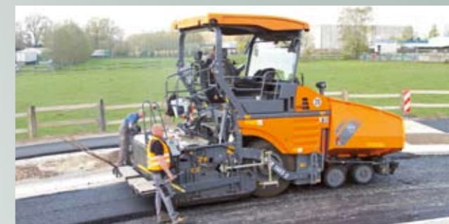
Construction de ronds-points
